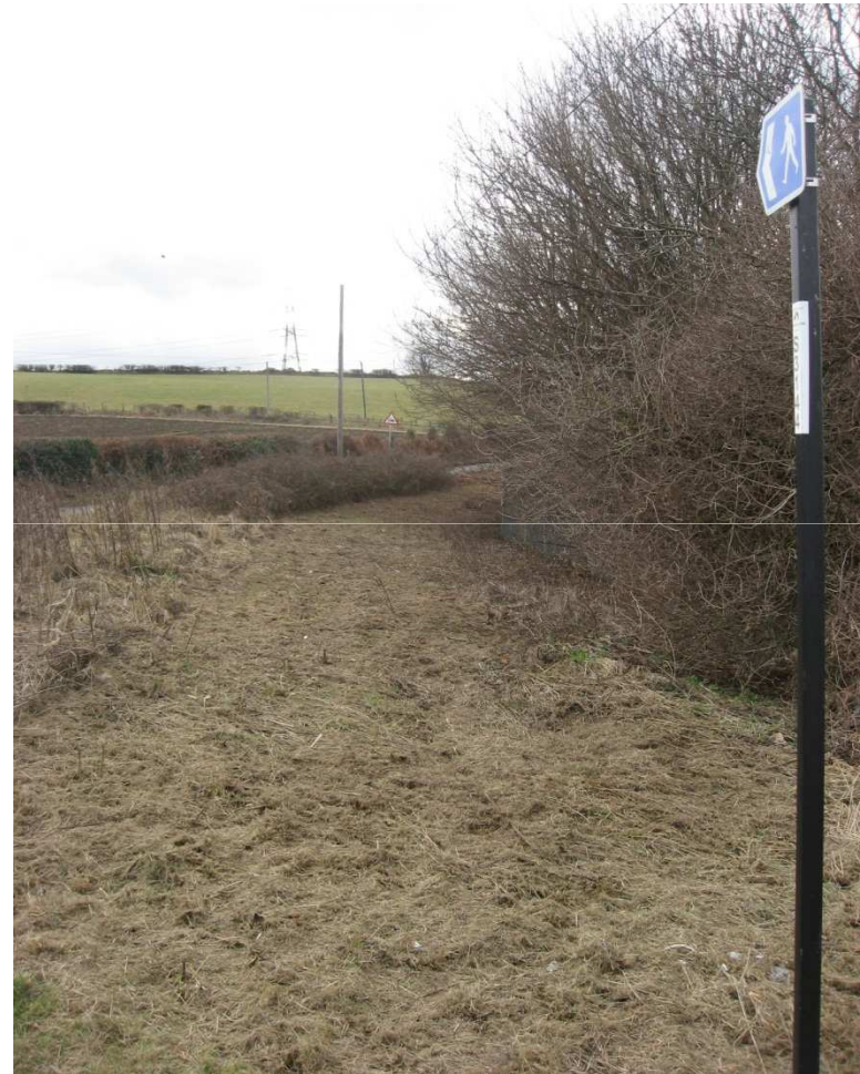
Verge clearance at Whiston
