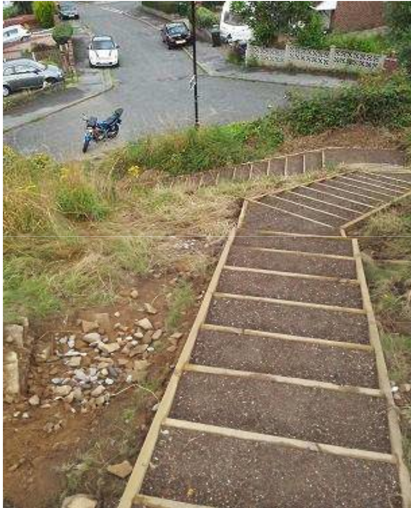
New steps – Kimberworth
