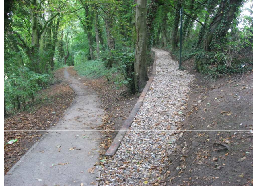
Path revetment at Maltby
